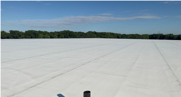
FIGURE 3: ENERGY-EFFICIENT WHITE TPO ROOFING
