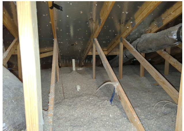
FIGURE 7: BLOWN-IN INSULATION
