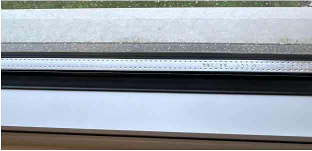
FIGURE 8: DOUBLE PANE LOW-E WINDOW
